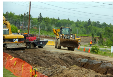
Membertou Infrastructure project
