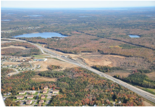
Membertou Highway Overpass Project
