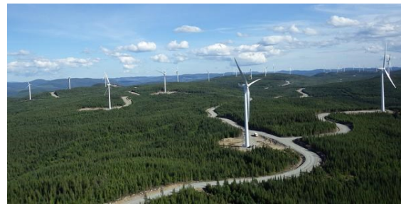
Rivière-du-Moulin Wind Farm
