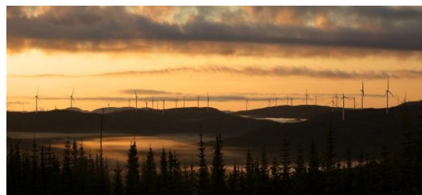
Rivière-du-Moulin Wind Farm
